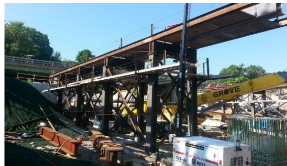
Figure C-95. Slide in of Bridge (Bhajandas et al. 2014)
