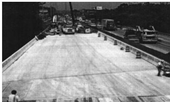
Figure C-34. Curing of New Deck (Bai, Burkett and Nash 2006)
