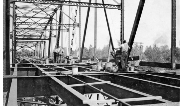
Figure C-66. Original Construction (Oregon DOT 1929)
