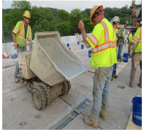
Figure C-116. LMC Placement (Ruzzi et al. n.d.)
