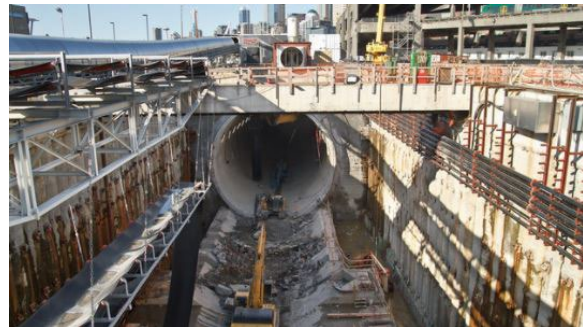
Figure C-10. Tunnel Construction (Washington State Department of Transportation 2020)
