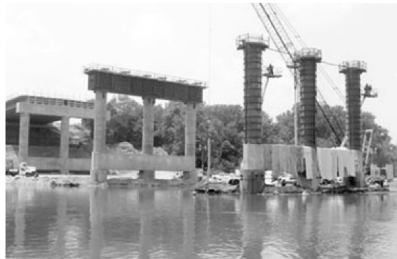
Figure C-52. Reconstruction of Piers (FHWA 2002)
