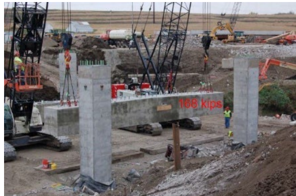
Figure C-101. Pier Cap Placement (Used with permission © Iowa Department of Transportation, Evans 2017)
