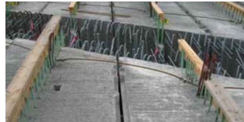
Figure C-124. Narrow Joints (Courtesy of PCI Journal, Khaleghi et al. 2012)
