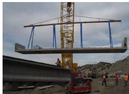
Figure C-106. Precast Slab Placement (Culmo 2011)
