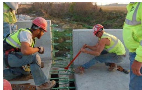
Figure C-102. Hairpin Fitting Challenge (Used with permission © Iowa Department of Transportation, Evans 2017)
