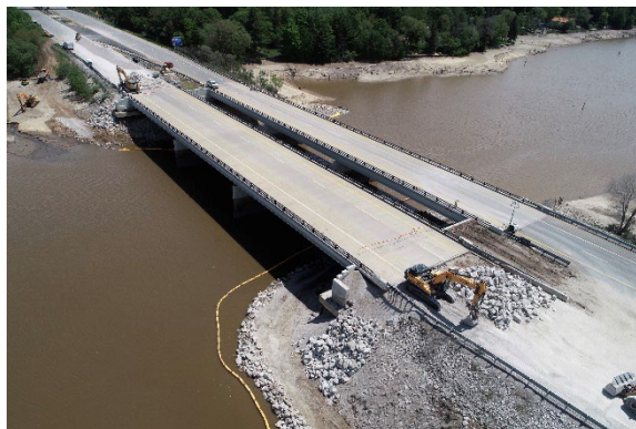
Figure C-21. Repairs to US-10 Bridge Approaches (Michigan Department of Transportation 2020)
