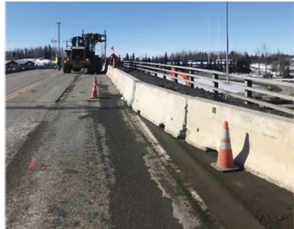
Figure C-44. Temporary Repair Clean Up 71106 (Levings & Murray 2019)
