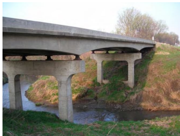
Figure C-98. Existing Bridge (Used with permission © Iowa Department of Transportation, Evans 2017)
