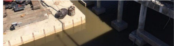
Figure C-26. Construction of New Spans (Tobia 2018)
