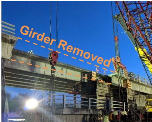
Figure C-45. Girder Removal 71104 (Levings & Murray 2019)
