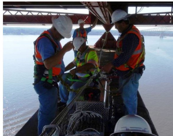
Figure C-55. Strain Gauge Installation and Wire Management (Courtesy of Sanya Watts, Watts 2013)
