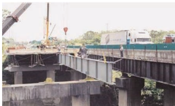
Figure C-33. Placement of New Girders (Bai and Kim 2007)
