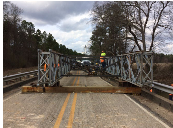
Figure C-19. Permanent Restoration (Courtesy of Heavy Bridge Maintenance, ARDOT) (A) Preparation for Jacking (B) Jacking System in Place (C) Launching of Bailey Bridge (D) Bailey Bridge Installed Across the Structure
