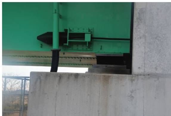
Figure C-6. Elastomeric Bridge No Damage (Kawashima & Matsuzaki 2012)
