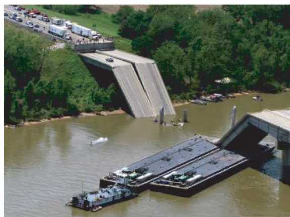
Figure C-51. Collapse of I-40 Webbers Bridge (Georgia Tech Research Corporation et al. 2012)
