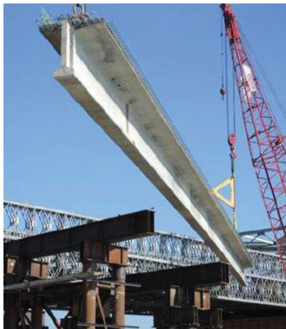
Figure C-72. Prestressed Girders Lifting into Place (Washington State DOT 2014)
