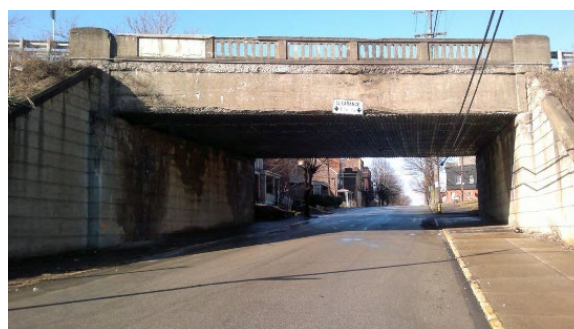
Figure C-112. Original Bridge (Ruzzi et al. n.d.)
