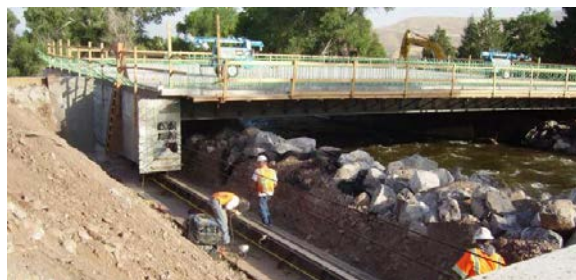
Figure C-107. Bridge Slide-In Installation (Culmo 2011)
