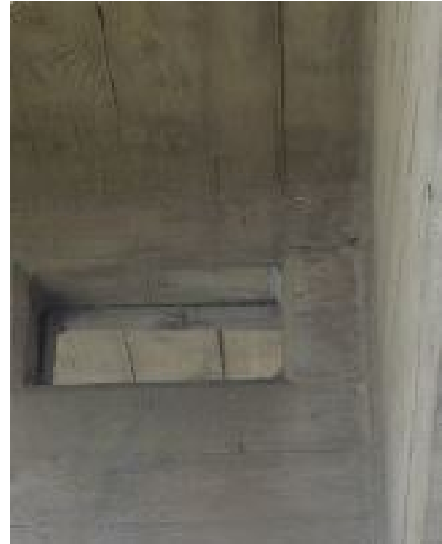
Figure C-30. Highway 11 Bridge Girder Opening (Chen et al. 2007 with funding from USGS)
