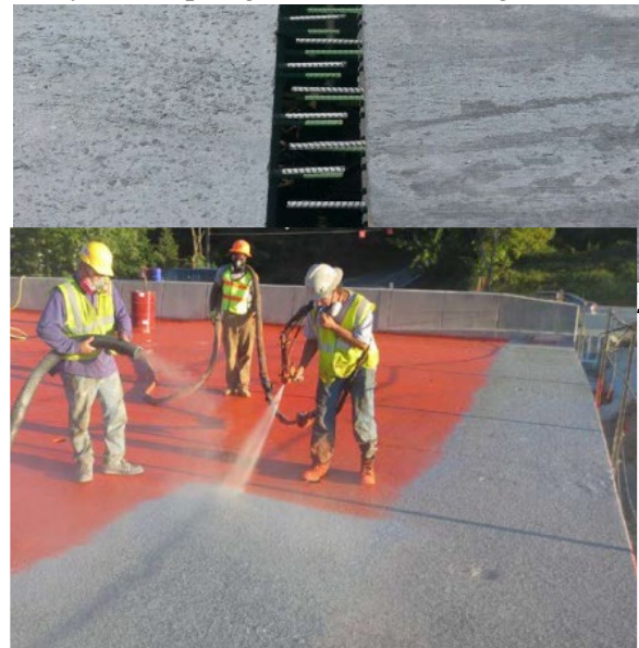
Figure C-93. Waterproofing Spray (Bhajandas et al. 2014)
