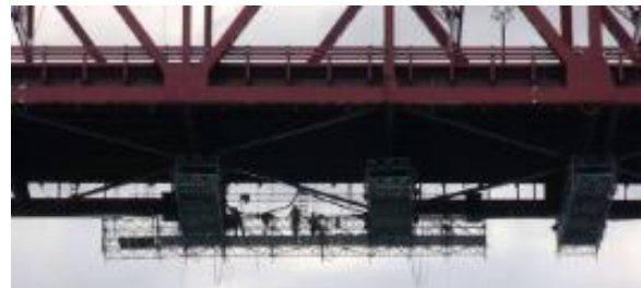
Figure C-57. Scaffolding on Mathews Bridge (Courtesy of Sanya Watts, Watts 2013)
