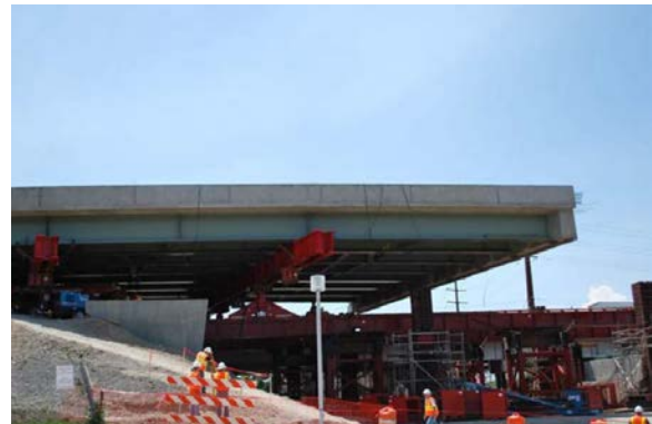
Figure C-110. SPMT on I-80 Bridge Replacement (Culmo 2011)
