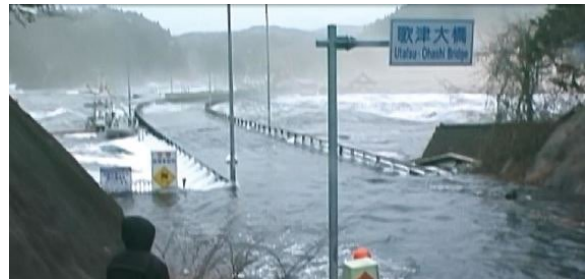
Figure C-2. Utatsu Bridge Flooded (Kawashima & Matsuzaki, 2012)
