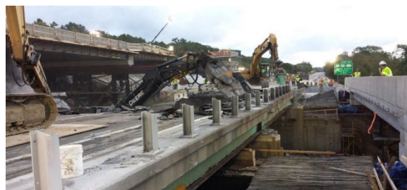
Figure C-89. Bridge Demolition (Bhajandas et al. 2014)
