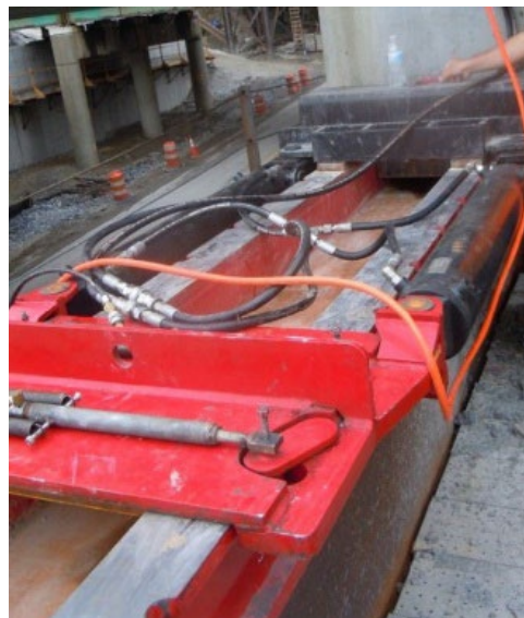
Figure C-94. Push Gripper Installation (Bhajandas et al. 2014)
