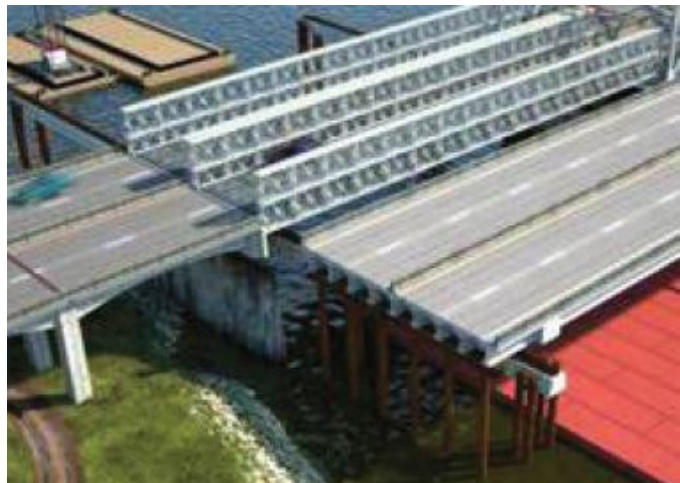
Figure C-71. Temporary modular bridge (Washington State DOT 2014)
