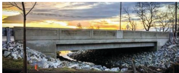
Figure C-77. A Bridge Built part of the P3 Project (Plenary Walsh Keystone Partners 2019)
