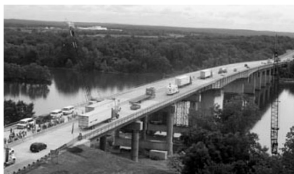
Figure C-53. Completed Repairs (FHWA 2012)
