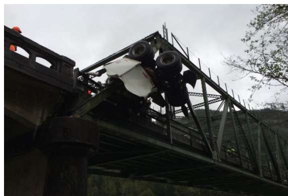
Figure C-65. Truck on Truss Member (Oregon DOT 2017)
