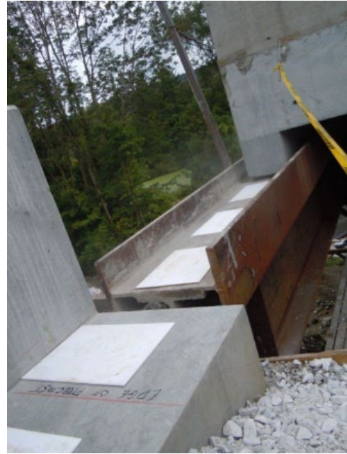
Figure C-97. Sliding of Approach into Place (Bhajandas et al. 2014)
