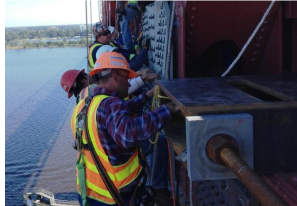
Figure C-61. Repairs made next to Temporary Chord (Courtesy of Sanya Watts, Watts 2013)
