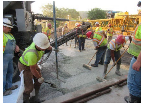
Figure C-117. UHPC Pouring of Joint (Ruzzi et al. n.d.)
