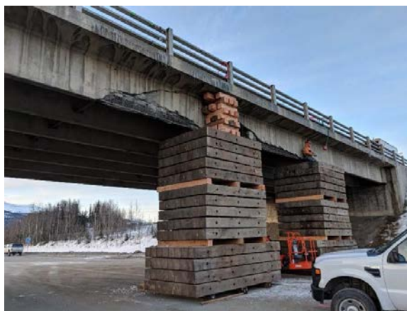
Figure C-43. Temporary Shoring Required for Girder Removal (Levings & Murray 2018)
