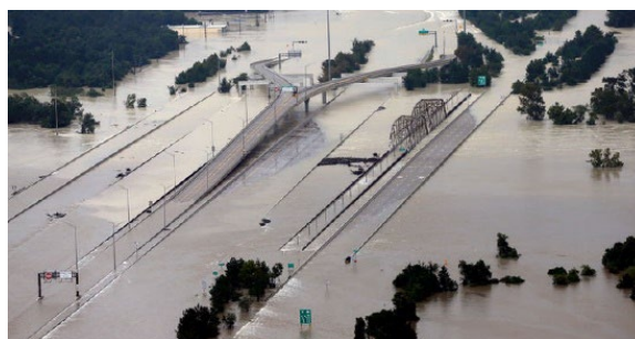
Figure C-22. San Jacinto River Flooding Over I-69 (Kirk 2018)
