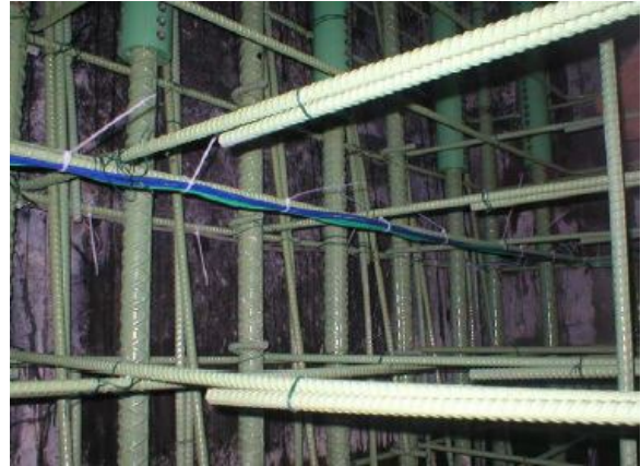
Figure C-84. in Gauges on the Reinforcement of Replacement Bridge (Collins et al. 2014)
