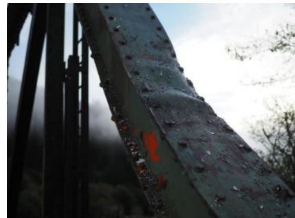
Figure C-68. Compression Member Buckling (Dobson 2017)
