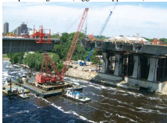
Figure C-82. Placement of Main Span Precast Segments (Figg & Phipps 2008)
