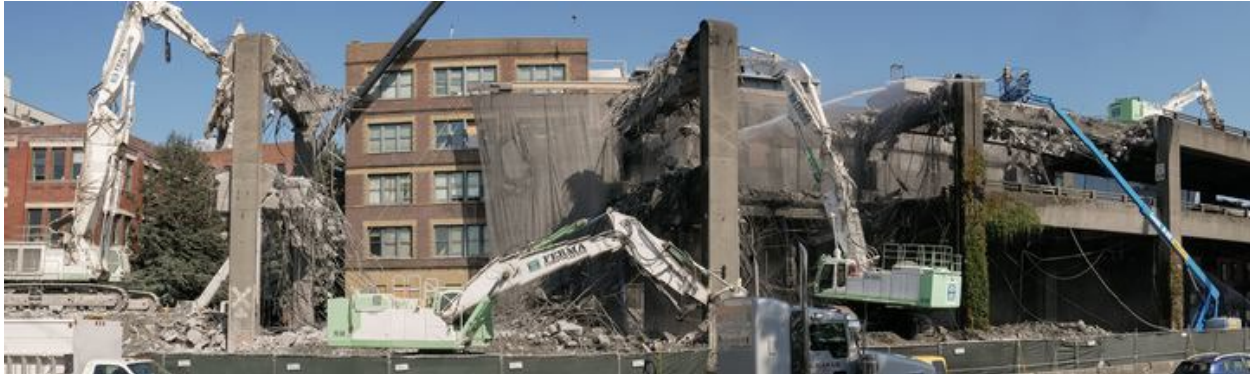
Figure C-12. Removal of Alaskan Way Viaduct (Washington State Department of Transportation 2018)
