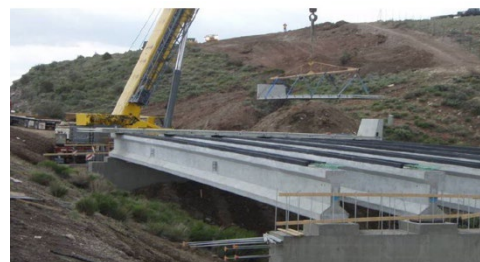
Figure C-105. Installation of Precast Element (Culmo 2011)
